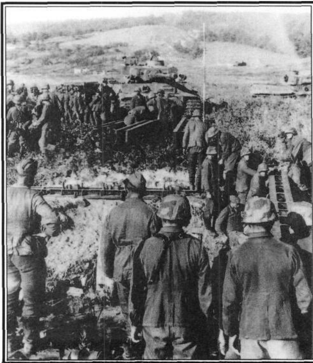
Left: An SS pioneer unit build an assault bridge across a ditch so that the waiting Tiger tanks can continue their advance. Such delays would inevitably give the Soviet defenders more time to prepare.
